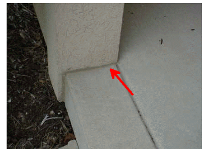
Seal or reseal EIFS to dissimilar materials.
