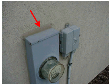
Reseal all utilities.
