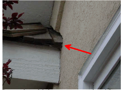
Secondary kickout returns should be installed.
