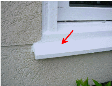
Sill vent flashing appears properly installed and is functioning.
