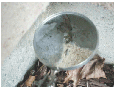
Yellow mesh is visible at terminations. (STO system)
