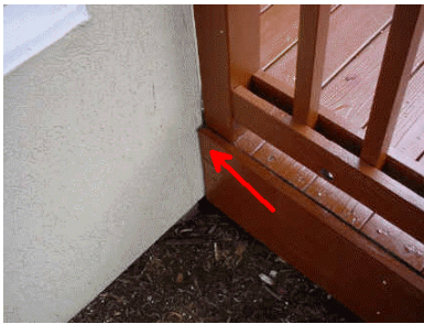
The deck is attached and sealed to the EIFS.
