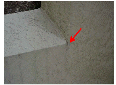
Repair cracking at corners on flat surfaces.
